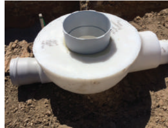
HALF POO PIT MAINTENANCE SHAFT
