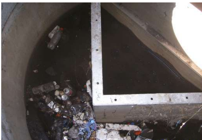
Trapped pollutants within the eco-BITE™ multi pollutant trap
